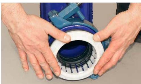
3. Insert NOVO-Grip® III ring into the pre-chamber.
