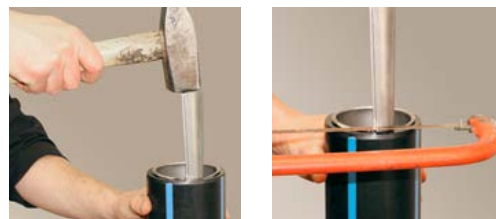
6. Drive the bracing wedge into the stabilising bush until it is tense. Cut off the protruding end of the bracing wedge.
