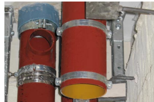
Before the fire test (below the ceiling)
