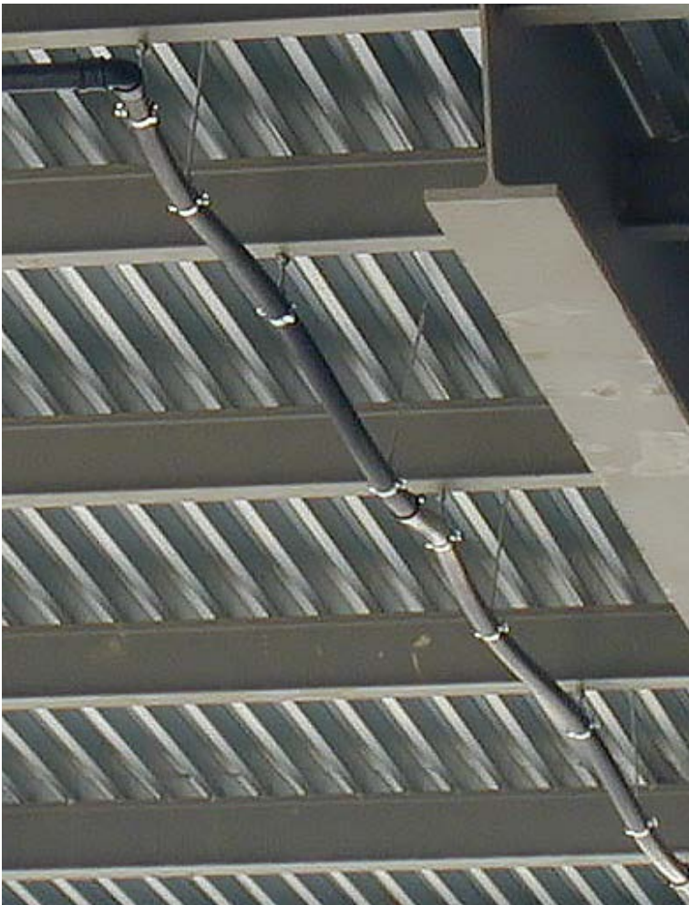
Problems with thermal length expansion: plastic pipes warped by heat below a hall roof – with Düker cast iron pipes that would not have happened!
